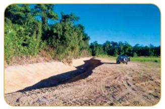
Example of detention basin/sediment trap. Note the steep batters, which required less production land. (Photo by Joe Rhodes).
