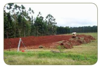
Sediment trap/sump under construction—bank in the background will be fenced and vegetated. Front batter has been made relatively flat to allow for grazing. (Photo by Joe Rhodes).
