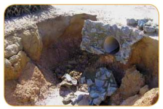
The incorrect design of this drainage outlet for the soil type and amount of runoff generated has resulted in bank collapse and the formation of a gully head which is retreating and contributing further sediment to the drainage network. (Photo by Ian Layden).
