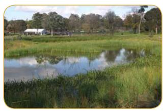
Constructed surface-flow wetland with emergent macrophytes around the edge
